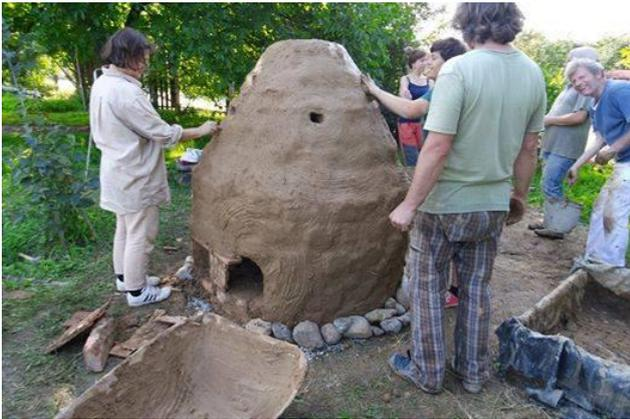
Construction of clay oven for pottery burning in made of the old earthen war and old bricks.
